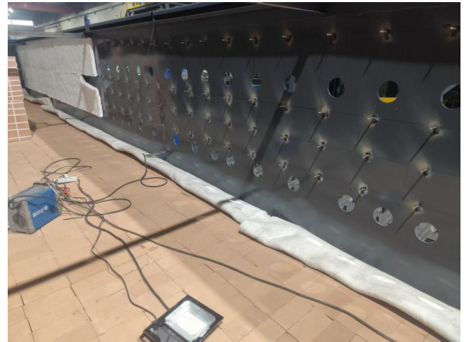
Step 4 : Install the module and the compensation blanket.
