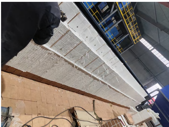
Step 5 : Cut the straps, and the module will expand.
