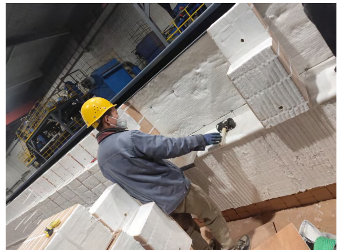
Step 6: Trim the module to give it a smooth and even appearance.
