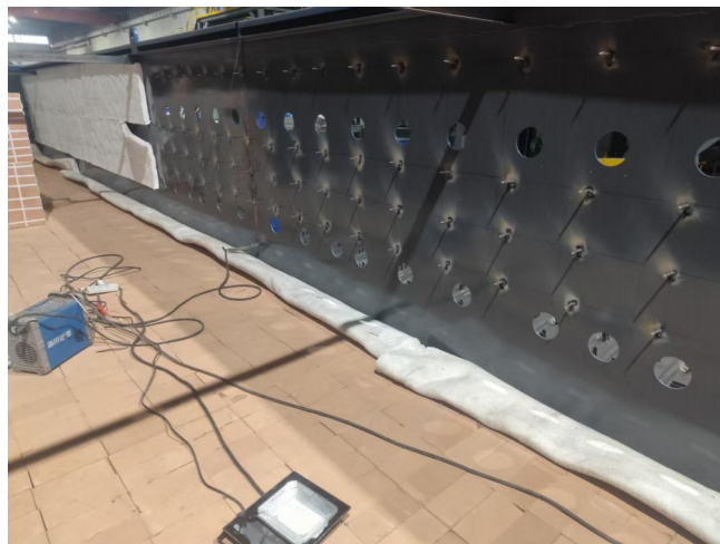
Step 5 : Cut the straps, and the module will expand.
